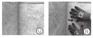
Use a damp rag or paper towel to clean off any sealant or adhesive that may have been squeezed onto the tile surface. When attaching accessories like coat hooks, mirrors or lighting fixtures that will carry a heavy load, drill a hole through tile and fasten to the framing inside the wall. Use a stud finder to locate framing before drilling through tiles.
