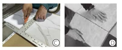
Cut tiles by scoring and snapping with a utility knife. (image C, D). This method may require sanding the snapped edges.
