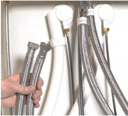
Connect to Shut Off Valves (not included)
