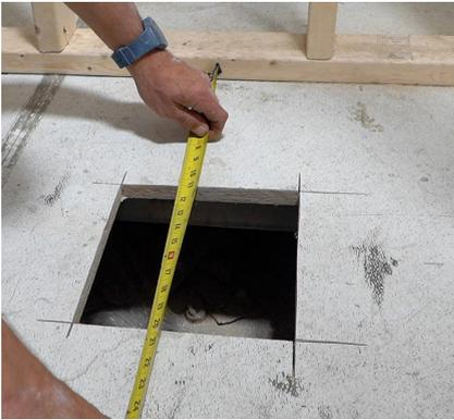
**1.** Measure carefully to determine the plumbing position and create plenty of access.
