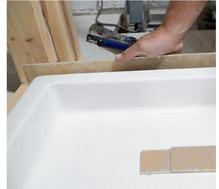
**9.** Place the flange carefully against the back side of the shower base making sure you have a good seal. Overlap the edge slightly so the flange will seal correctly at the corners.
