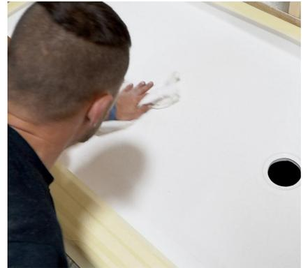
**6.** Clean the base thoroughly before placing the cardboard protection plate down.
