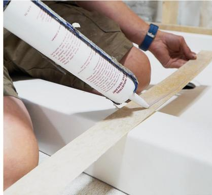
**14.** Run a bead of 100% silicone caulk on the lower third of the flange.
