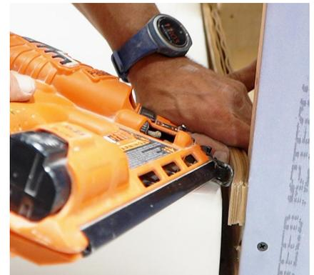
**12.** You may require shims for a tight fit for the flanges. Use as many cardboard shims as needed to secure a tight fit. Then, tack them into place.
