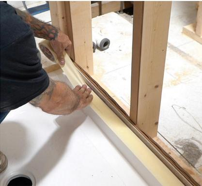
**4.** Mask off the rim of the shower base to protect it from dirt, scratches, and other potential damage.
