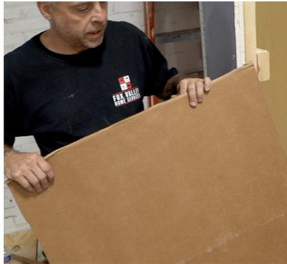
**5.** Cut a piece of cardboard to fit it in the pan for complete protection of the base.
