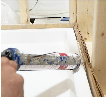
**13.** Place a bead of 100% silicone caulk on the cardboard shim so it seals tightly against the back side of the flange.
