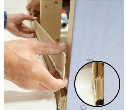
**15.** Slide the shims carefully into position leaving one to one and a half inches of clearance from the top of the base.
