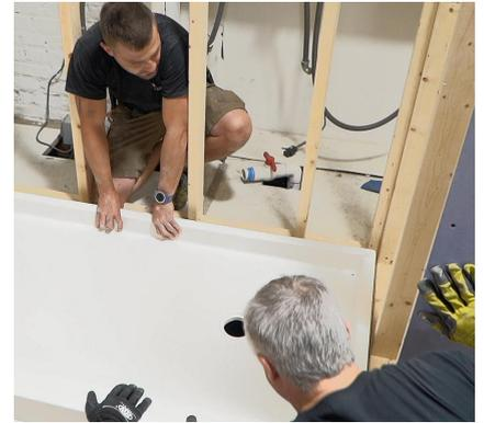
**3.** Push the shower base carefully in leaving about a half inch clearance from the back wall to accommodate flanges.
