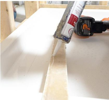
**16.** Run another bead of 100% silicone caulk concealing the base and the flange. Make sure there are no gaps in your bead of silicone.
