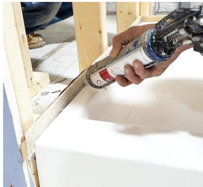
**17.** Repeat the same process for the other side using the proper amount of shims and sealing them with a bead of 100% silicone caulk.
