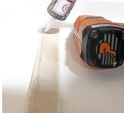
**8.** Run a bead of silicone caulk down the lower third of the flange keeping about an inch to an inch and a half above the shower base.
